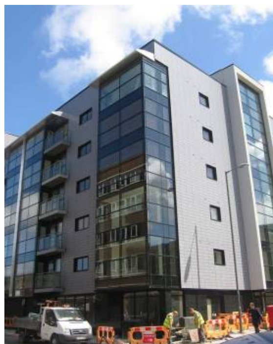
Hamilton House, Pall Mall, nearing completion in May 2009
