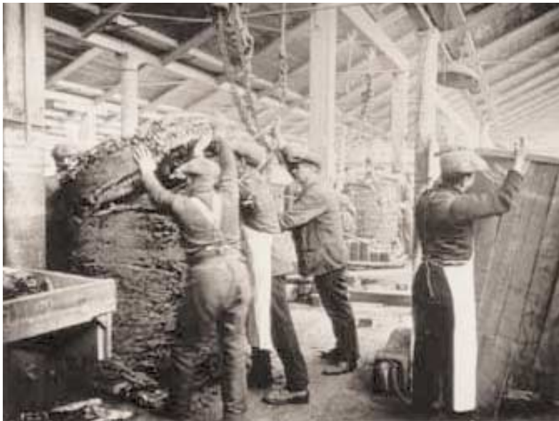
Stanley Dock Warehouse, men weighing Tobacco leaf 1918 - E. Chambre Hardman © E Chambre Hardman Trust
